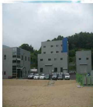
Front view of plant
